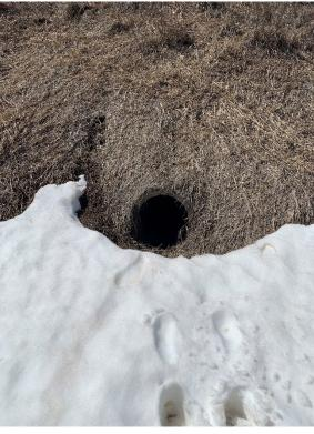
Culverts found in area of major derailment collapsed and plugged not allowing water to drain under roadbed.
